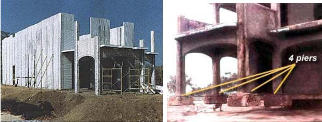
The building, left high and (not so) dry, with no support from below, lost none of its tensile integrity. The builder needed only to pour concrete footings under the existing columns, backfill with dirt, and the owners of the structure can rest assured that their homes will stand safely throughout whatever nature may have planned for the future.
